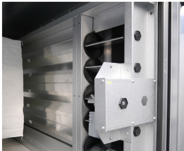
Damper bypass in unitate.
